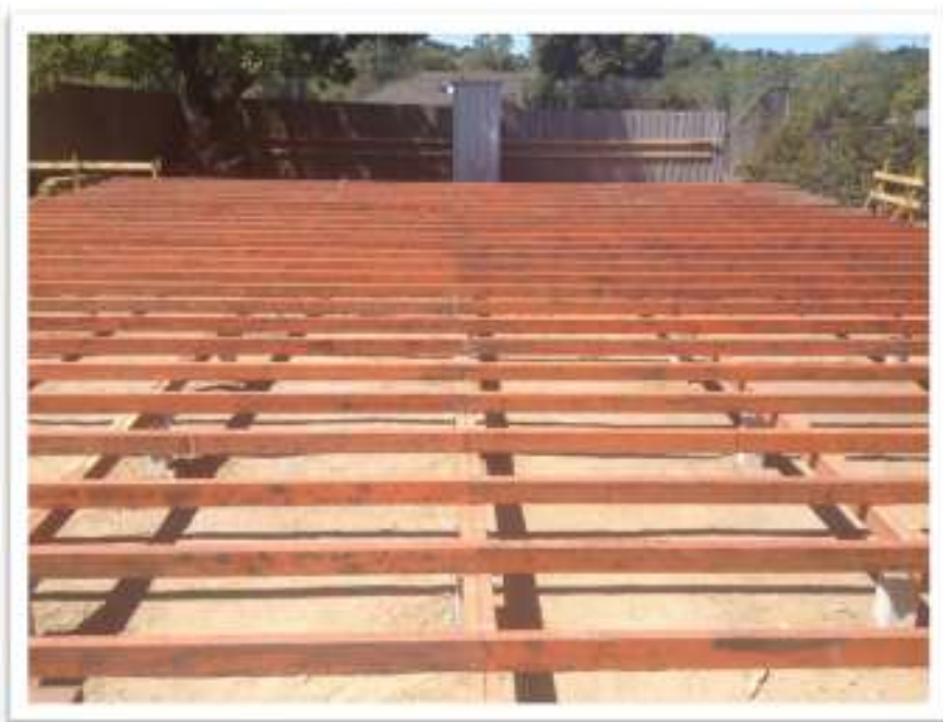
A photographic example of open timber bearer and joists.
